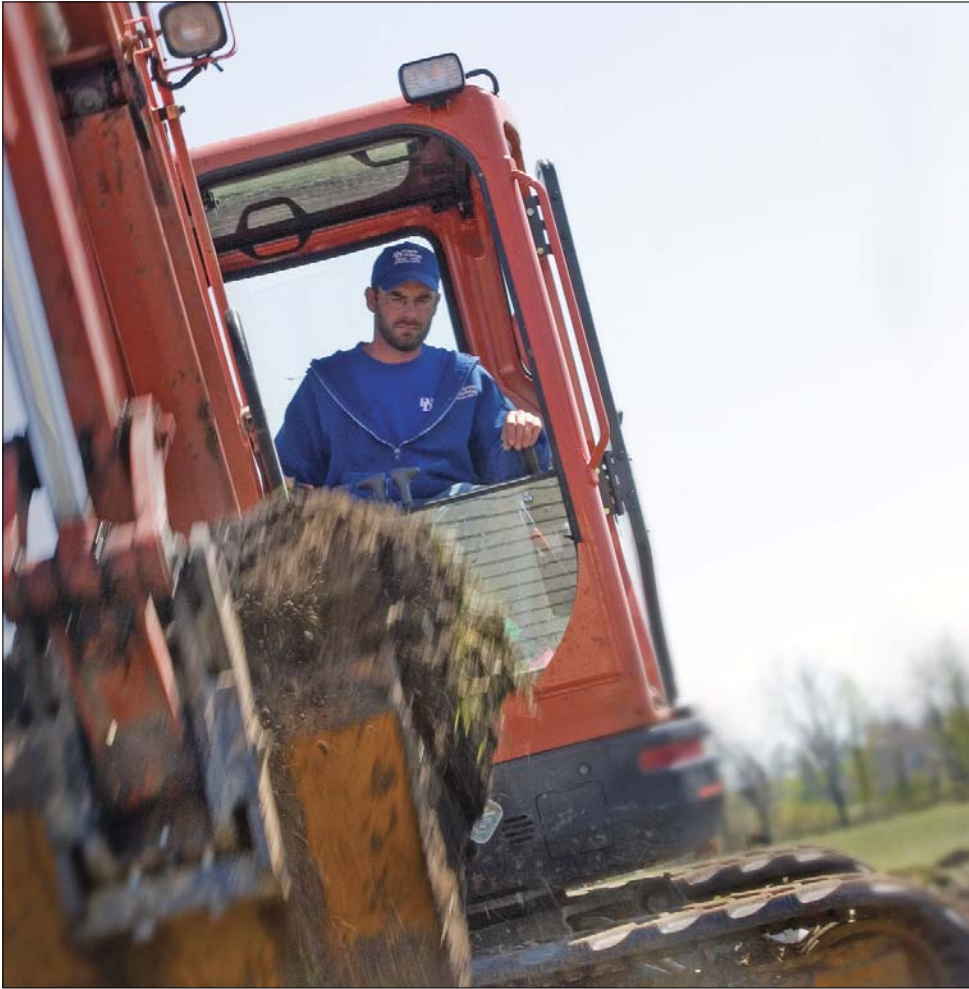
↑ Patrick Dittmer operates an excavator.
