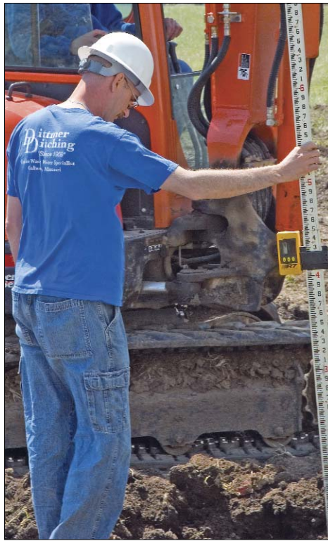
↑ Matthew Dittmer checks the grade for placement of drainfield chamber.
